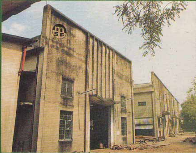
Working Sheds of the Factory
